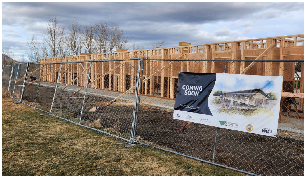
New construction of MT Wild Avian Building. Photo by Sue Jackson
